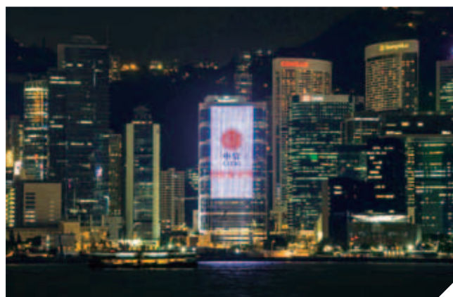
LED light decoration (35m W x 91m H) on the northern façade of CITIC Tower
