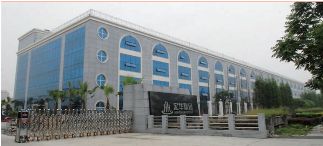
Honghua's headquarters located at the Technology Park, Jinniu District, Chengdu
