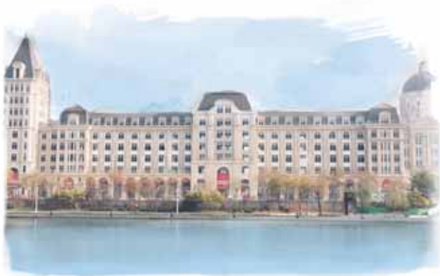
City Plaza (Tianjin)
