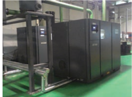
Vacuum pump transformation projects of Hangzhou Company
