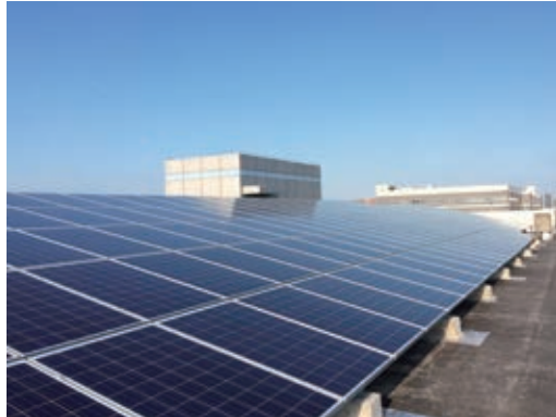
Photovoltaic power generating projects
