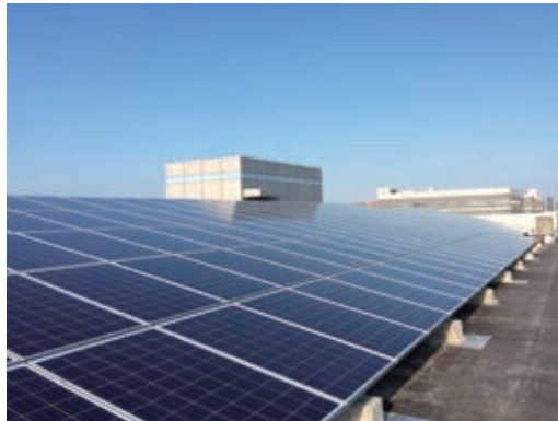
Photovoltaic power generating projects
