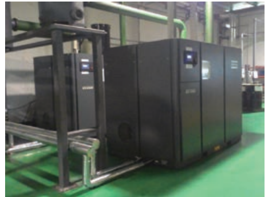
Vacuum pump transformation projects of Hangzhou Company
