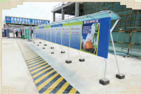
A bulletin board was set up at Yuzhou Prince Lakeshire project site in Bengbu to remind employees of safety issues.
