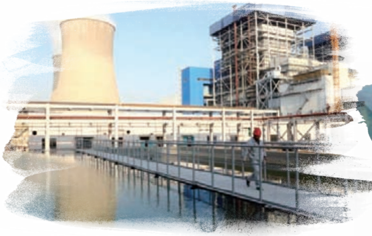
Photo: Installation of raw water treatment system to reduce water consumption
