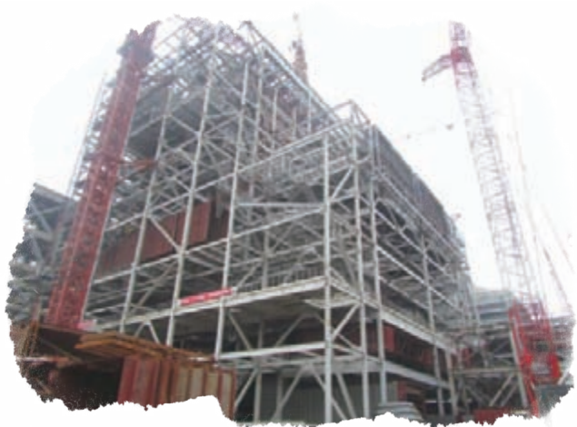
Photo: Upgrade of denitration system
