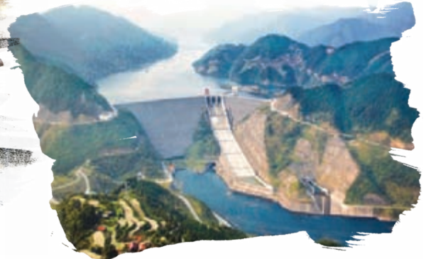
Photo: Floodgate of San Ban Xi Power Plant retrieves 1,961 million cubic metres of water that enables additional power generation of 565,000 MWh.
