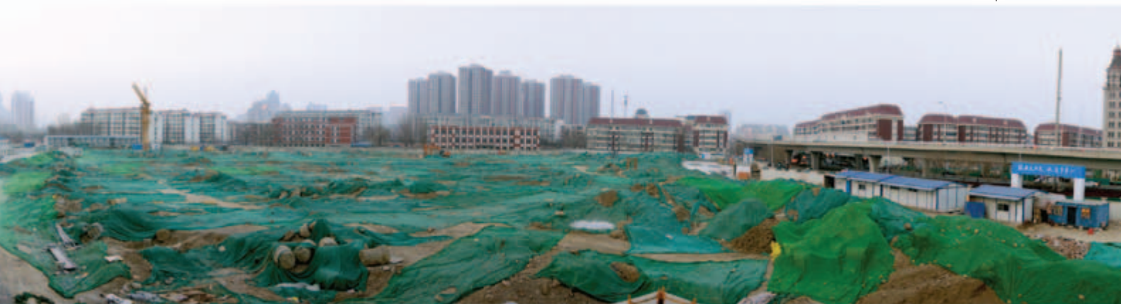
■ Piling works for the composite development in Tianjin already completed
