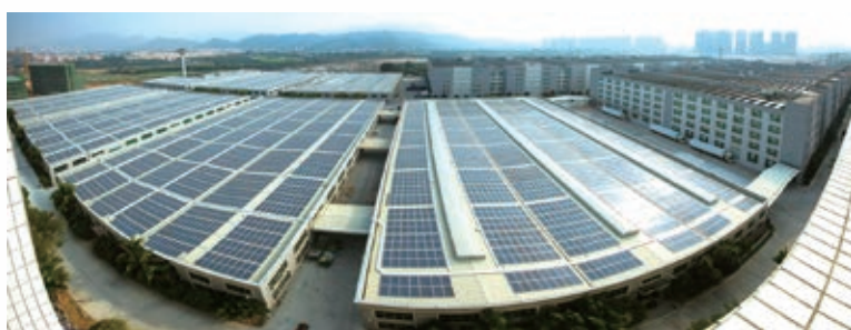
(Photo caption) Huizhou Plant rooftop solar panels
