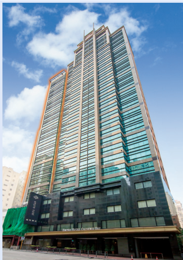
Empire Hotel Causeway Bay and the adjacent new hotel
