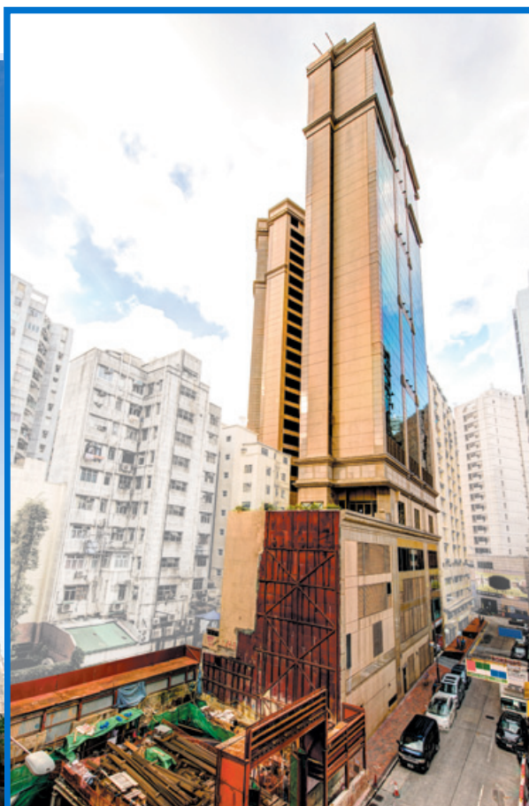
Empire Hotel Kowloon and the adjacent new hotel development
