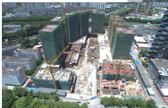
Enterprise Square - construction works in progress
