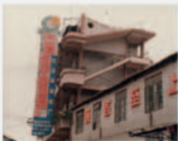
90's The exterior of Dongpeng Ceramic Central Factory
