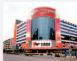
2005 The exterior of Dongpeng Building (東鵬大廈)
