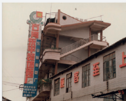
90's The exterior of Dongpeng Ceramic Central Factory
