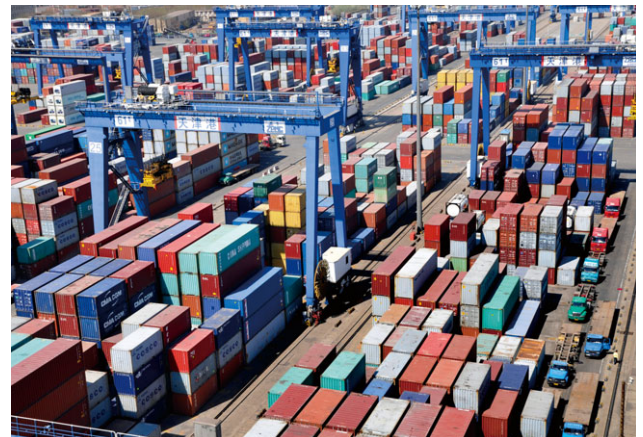
Tianjin Five Continents International Container Terminal
