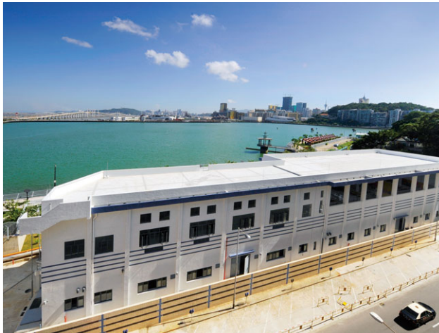
Macau Water Plant
