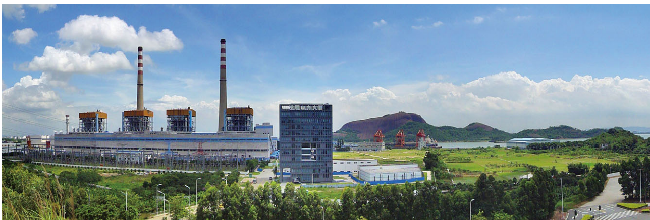
Zhujiang Power Stations
