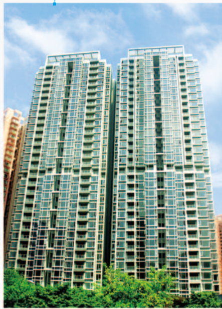
Guangzhou Eastern Place Phase V
