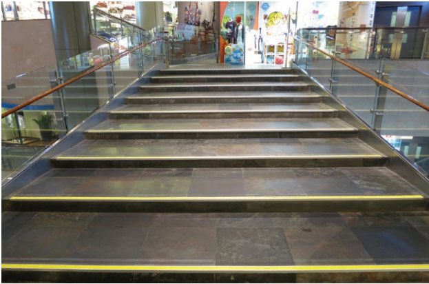
Non-slip Nosing to Staircase
