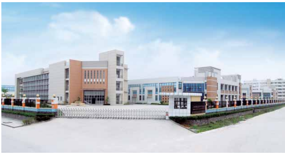
Aluminum foil factory in Qingyuan of the PRC 中國清遠鋁箔廠房
