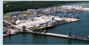
Vesta Terminal Tallinn, Estonia, Europe 35 storage tanks Storage capacity: 405,600 m 3
