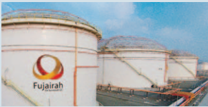
Fujairah Oil Terminal, United Arab Emirates, Middle East 34 storage tanks Storage capacity: 1.155mm m 3
