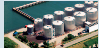
Vesta Terminal Flushing, Holland, Europe 27 storage tanks Storage capacity: 388,500 m 3
