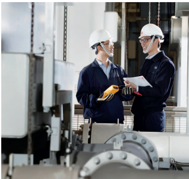
Systematic equipment inspection and maintenance ensure supply reliability.
