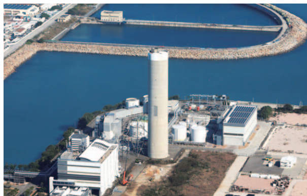
Construction commences on HK Electric's L10 gas-fired unit.
