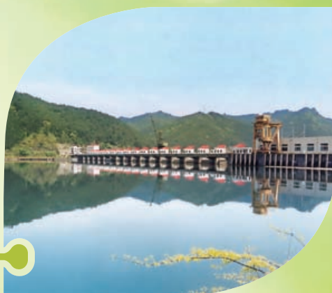
Fujian Shaxikou Hydro-electric Power Plant
