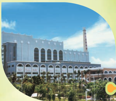
Haikou Waste Incineration Power Plant
