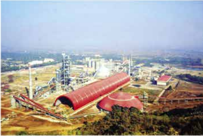
The cement and clinker production line with a capacity of 5,000t/d of Myanmar Conch has been put into operation.
