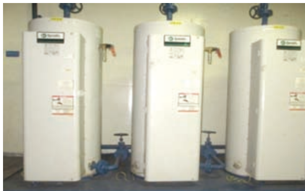
Boilers after replacement
