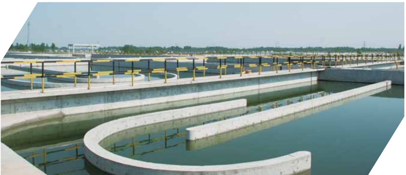
The largest sewage treatment plant in Hunan, construction contracted by the Company
