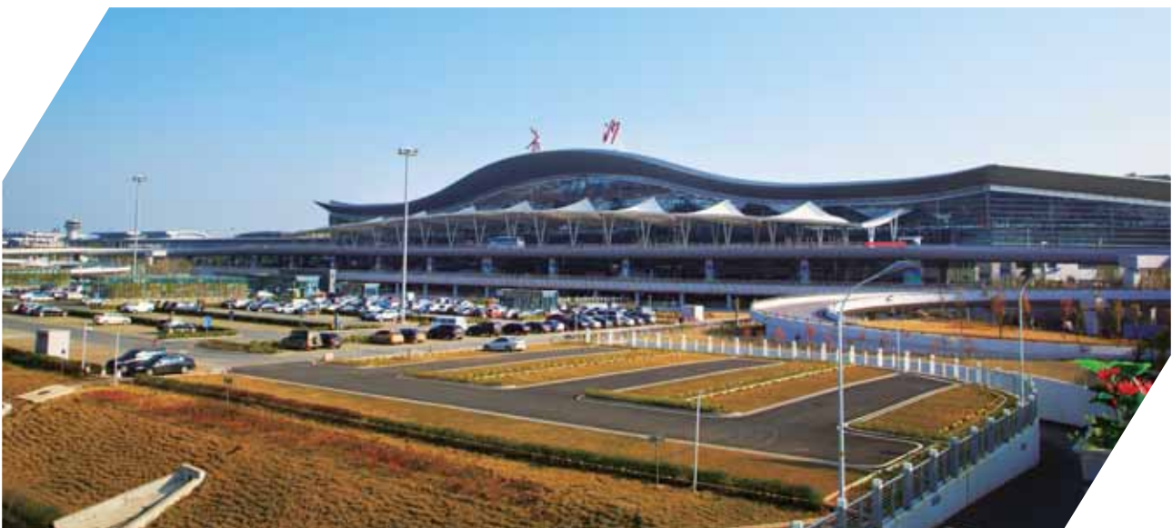
Engineering of power station for provision of air-conditioning, heating and electricity in Huanghua Airport, construction contracted by the Company
