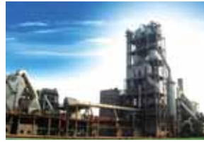
New dry cement production line (Construction material industry)
