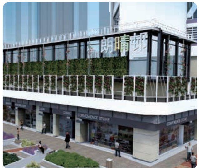
Public Rental Housing Development in Yuen Long (Long Ching Estate)
