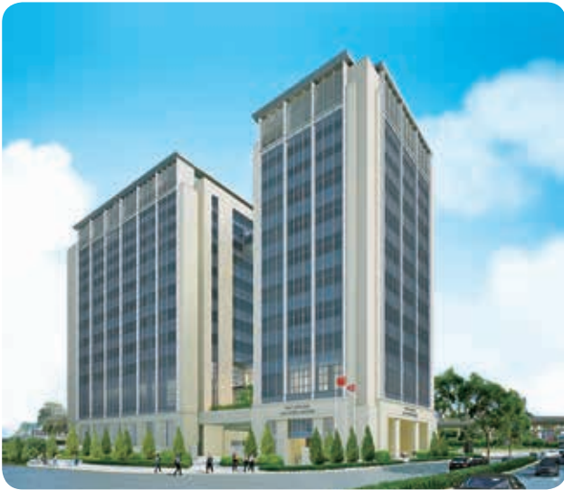
West Kowloon Law Courts Building
