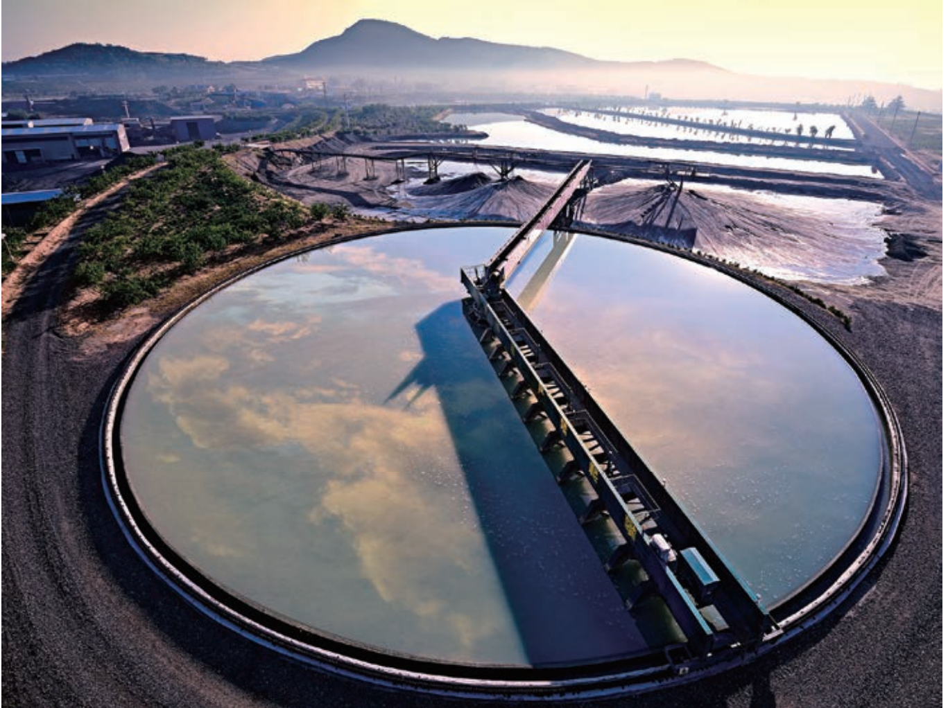
Patented tailing dam dry discharge system (Yangzhuang Iron Mine)
