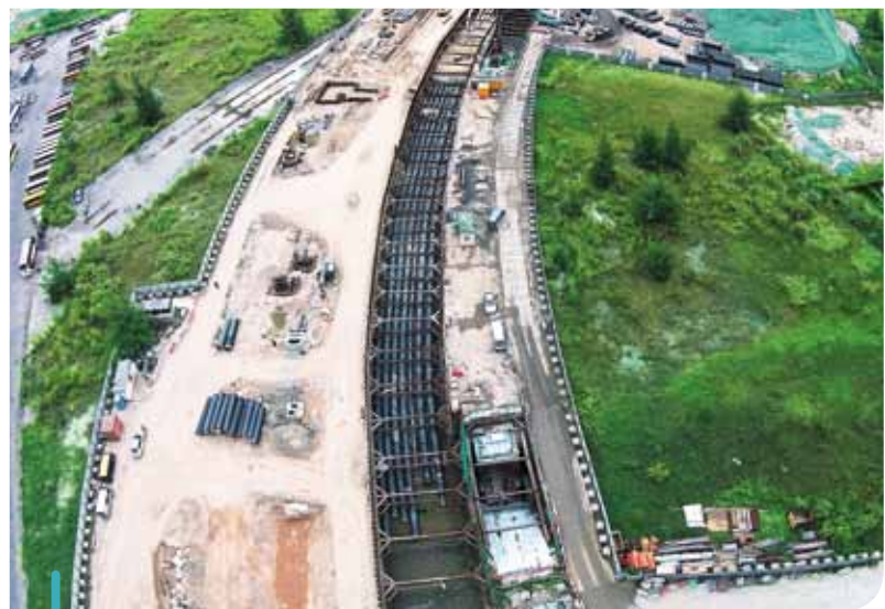
The construction of an underground seawater cooling system and associated works in the Kai Tak Development Area by U-Tech is progressing well.
