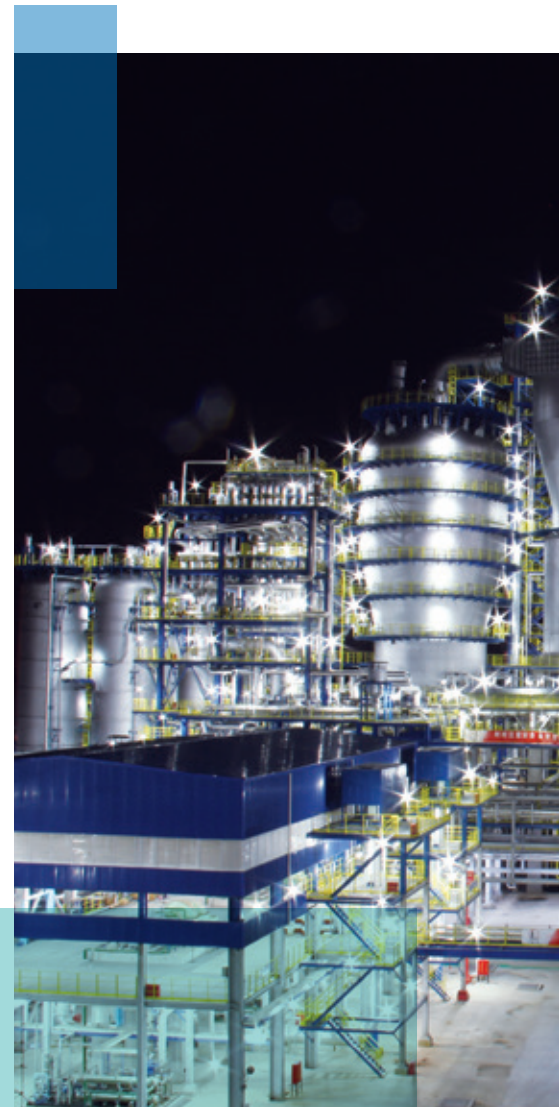
The panorama of MTO production facility (as at Mid-August 2014)
