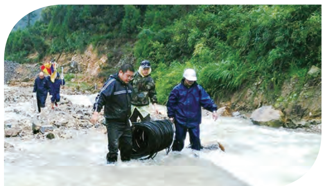
Post-disaster restoration of base station
