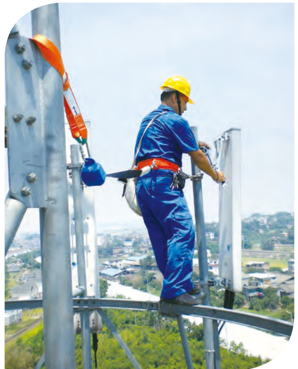
The Group undertook 4G network construction projects
