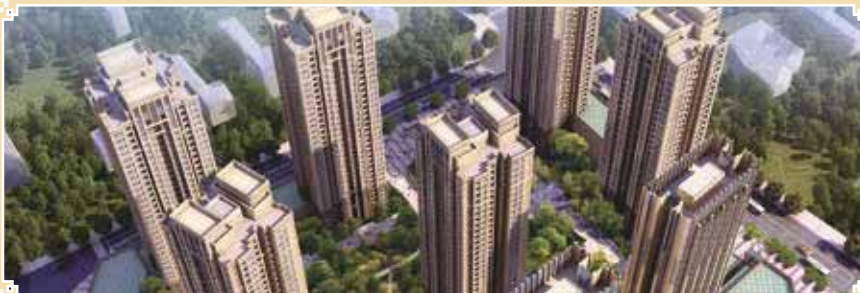
Chongqing Panlong Jinmao Residence
