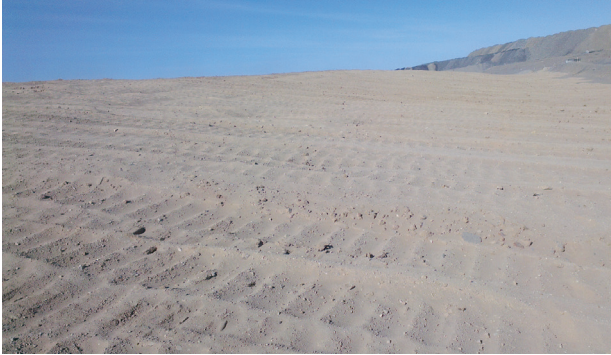
Preparation of topsoil stockpile for vegetation
