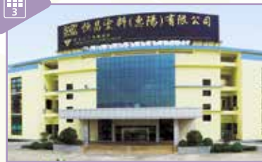
位於廣東惠州的塗料廠房 The coatings plant in Huizhou, Guangdong
