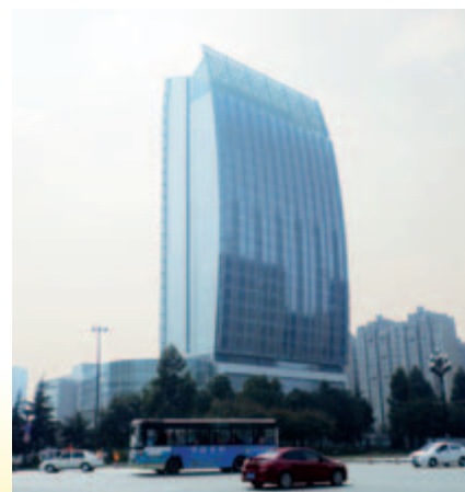
■ Regal Xindu Hotel, a five-star hotel in the first stage of the composite development – superstructure works completed
