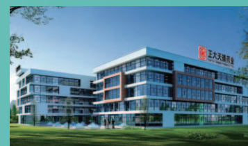
CT Tianqing's R&D Centre
