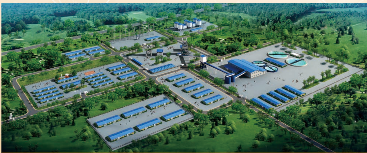
A bird view of the mining and processing project of Chambishi Southeast Mine
