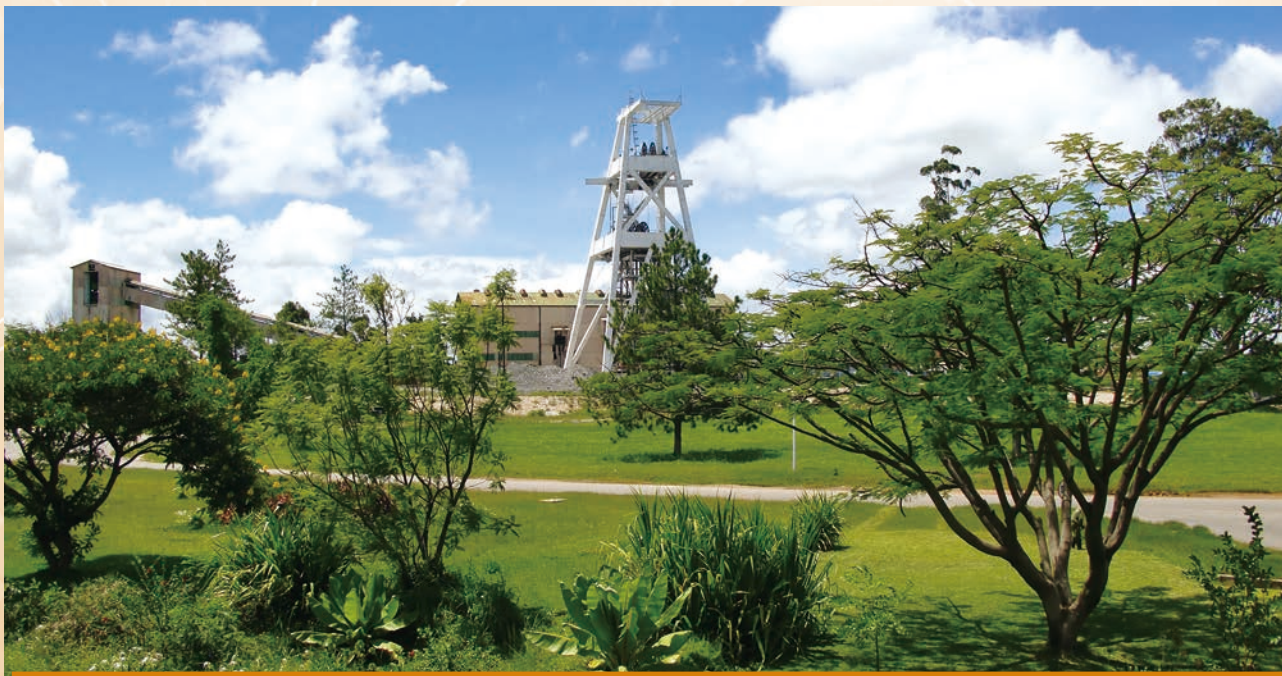
Main shaft of Chambishi Copper Mine
