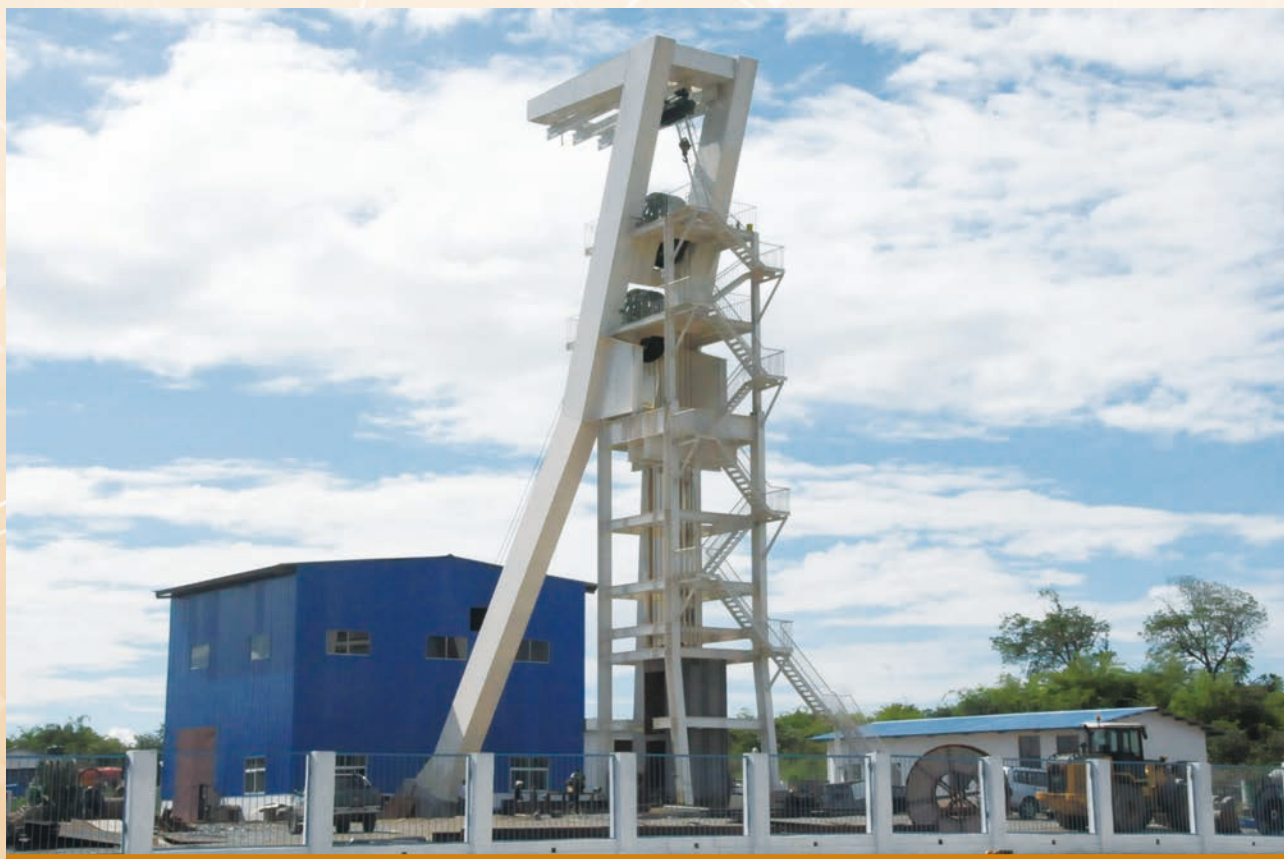
Central auxiliary shaft of Chambishi West Mine
