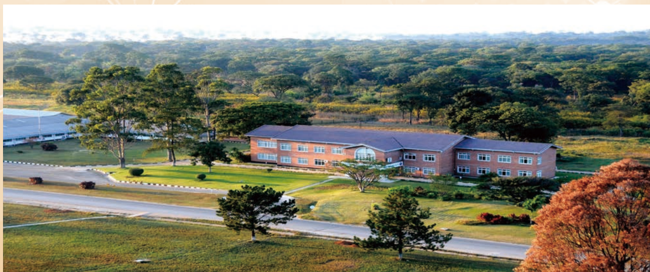
Central office building of NFCA in the green bush
