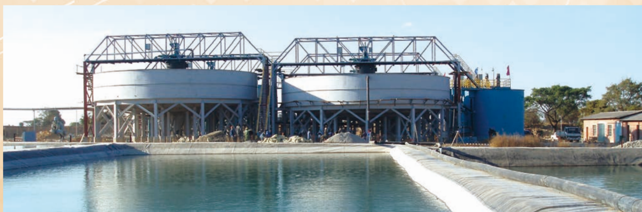
Settling pond for leaching
