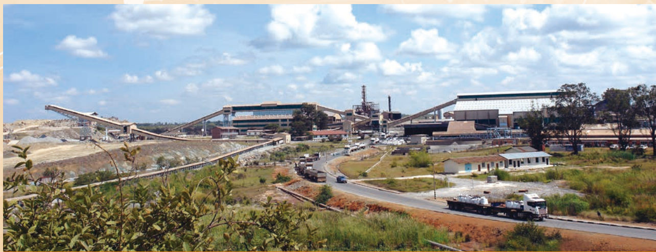
Panorama of Chambishi Copper Mine processing plant
