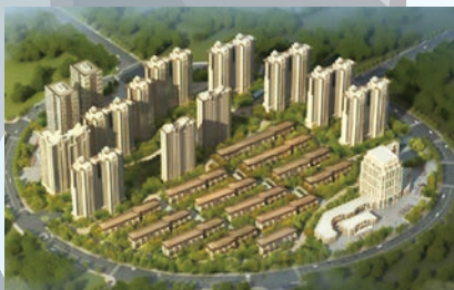
Bird's-eye view of Langfang Longhe New District Project
