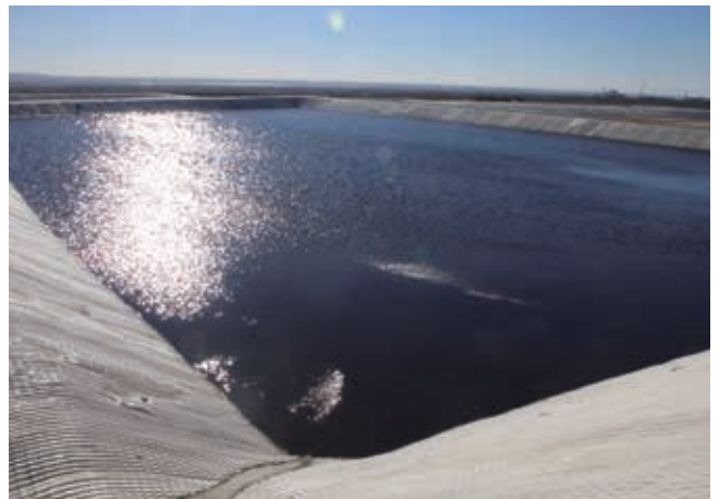
Waste water treatment
