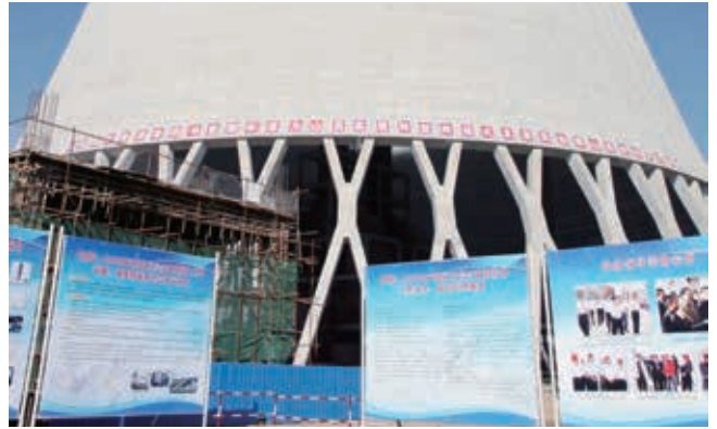
Desulphurization and denitration renovation works of power plant
