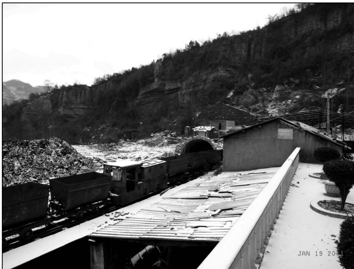
Figure 13-14: View of Tiziyan Mine in 2011
