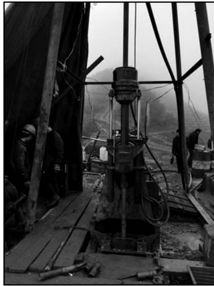
Figure 9-1: Drilling Rig of 2014 Drilling Programme
