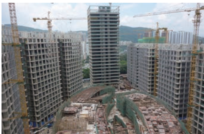
Enterprise Square – construction works in progress
