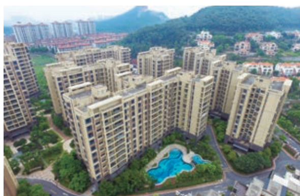
High-rise apartments under Phase 1 of Metropolitan Oasis
