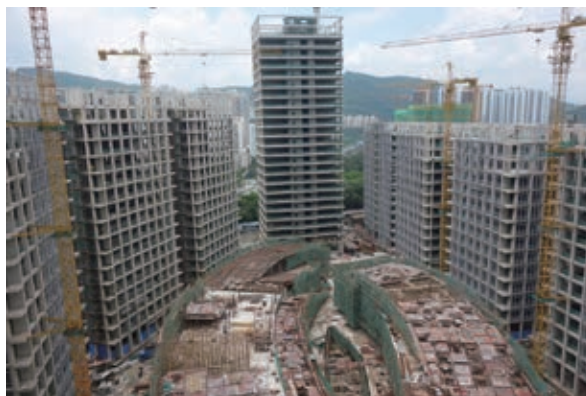
Enterprise Square – construction works in progress
