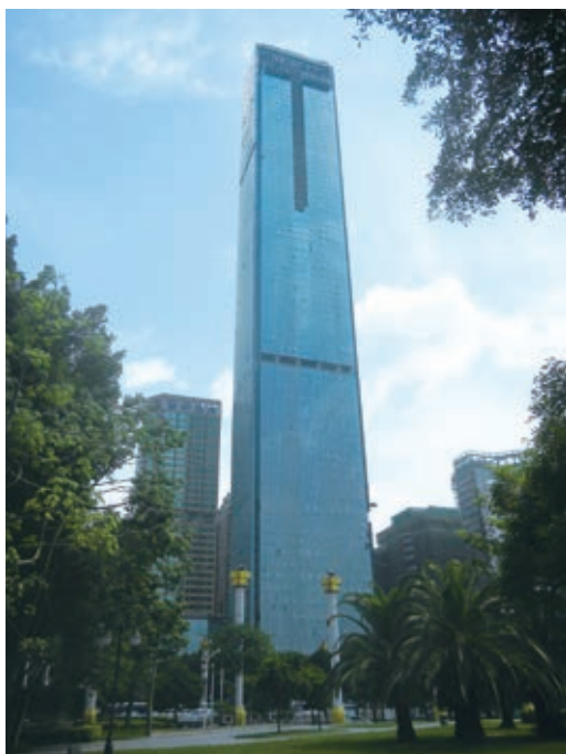
Hon Kwok City Commercial Centre – construction works in progress
