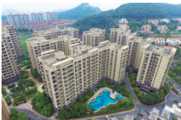
High-rise apartments under Phase 1 of Metropolitan Oasis
