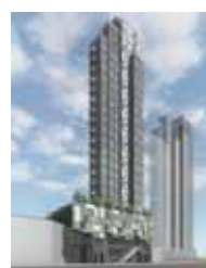
A development site at Tai Wai, Hong Kong
