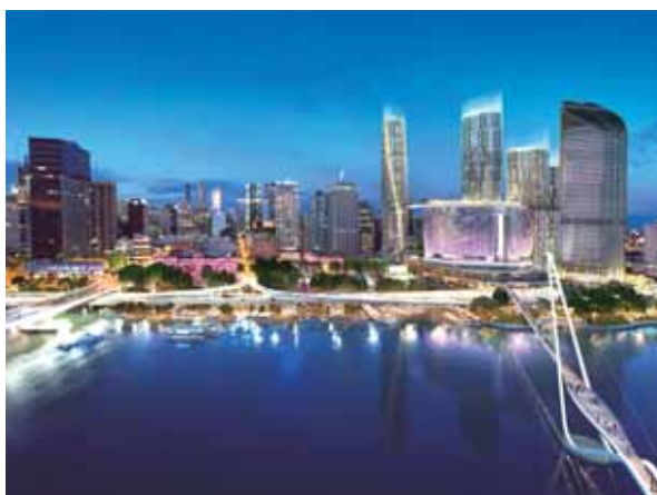
Queen's Wharf Brisbane Project, Australia
