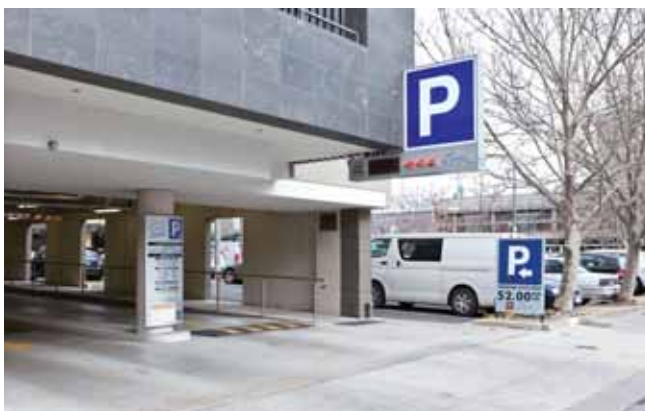
Car Park Operation
