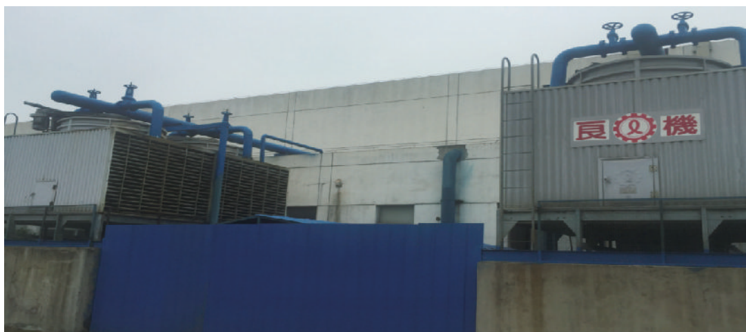
Cooling water circulation system
