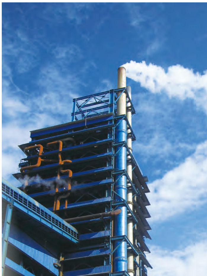
ISA furnace of copper smelting company
