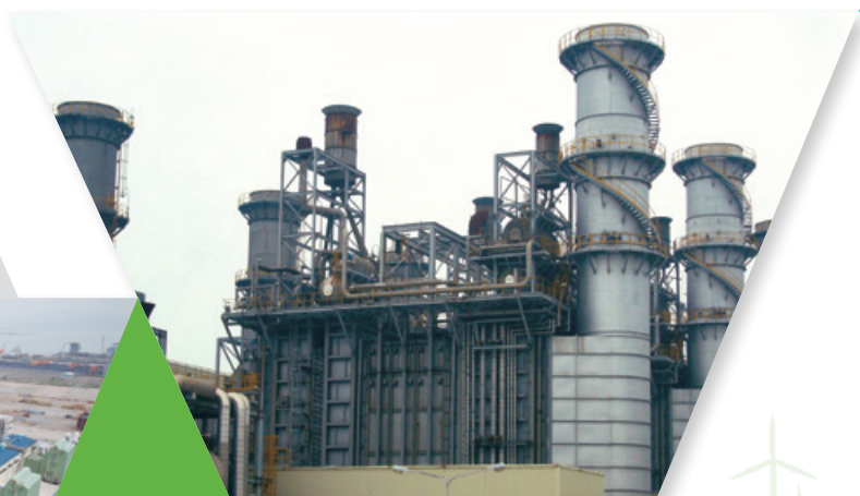
Daesan Oil-fired Project (Phase I)
