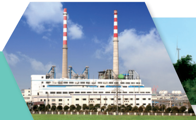
Nantong Cogen Project
