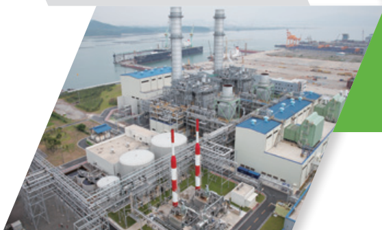
Yulchon Gas-fired Project (Phase II)
