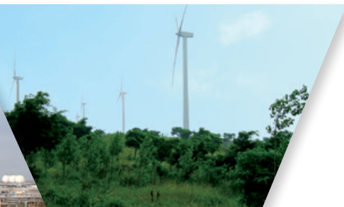
Taipingshan Wind Power Project (Phase I)
