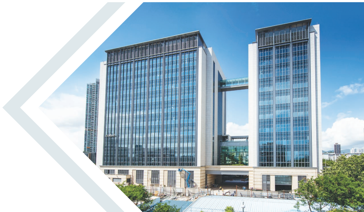
West Kowloon Law Courts Building
