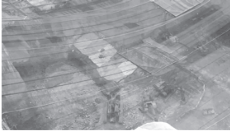
Rock excavation works by surface drill and blast method
