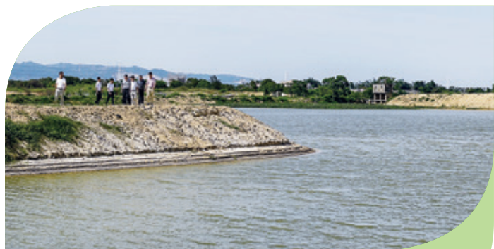
Completion of impounding after construction
