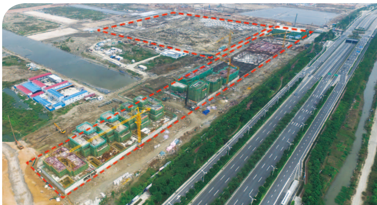
Hengqin Novotown Project Phase I
