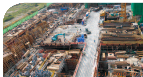
Latest construction progress of Alto Residences
