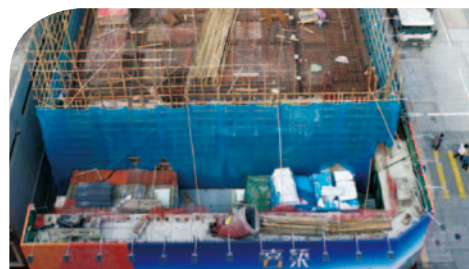
Latest construction progress of 93 Pau Chung Street
