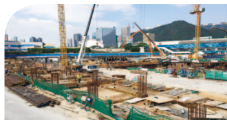
Latest construction progress of Ocean Hotel project
