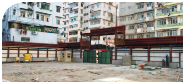
Latest construction progress of Ki Lung Street project
