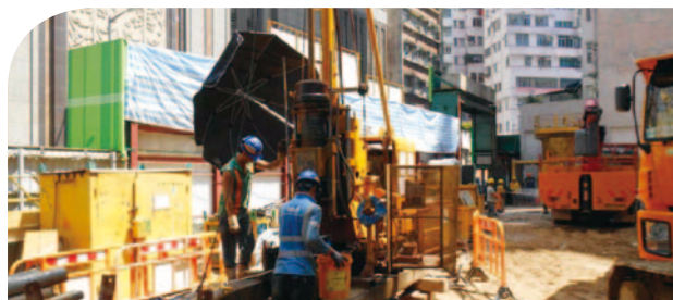
Latest construction progress of Sai Wan Ho Street project
