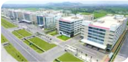
First Vietnam Facility 首家越南廠
